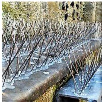
Under the expert instruction of Iain Frearson, our Church Architect, Steve Austwick and Chris Mitchell of H Austwick Lead and Copper Roofing, Stow-cum-Quy, are hard at work fitting spikes on ledges and placing spiked wire cages in roof gutters to stop pigeons from nesting in these spaces. Preliminary clearance work was carried out between July and December 2018 by Soham-based firm Peter Saunders Builders and paid for by a generous donation from the Ivy Mary Mefie Deceased Charitable Fund. We
